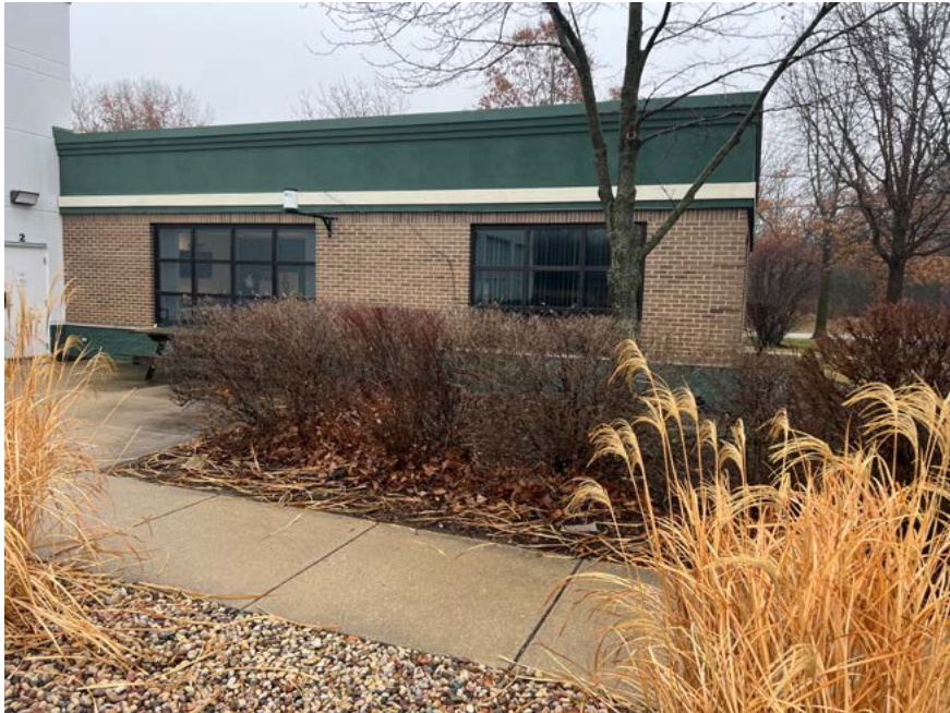
SE Entrance terminata at building
