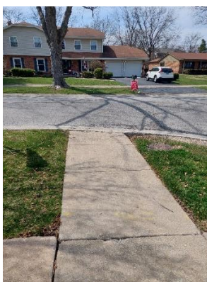
Remove South Sidewalk Ramp with No Receiving Ramp
