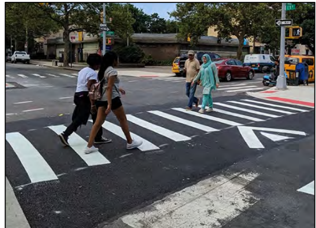
Figure 5-23. Raised crosswalk example
