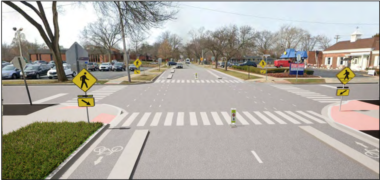
Figure 5-6. Flossmoor Road at Douglas Avenue, looking west
